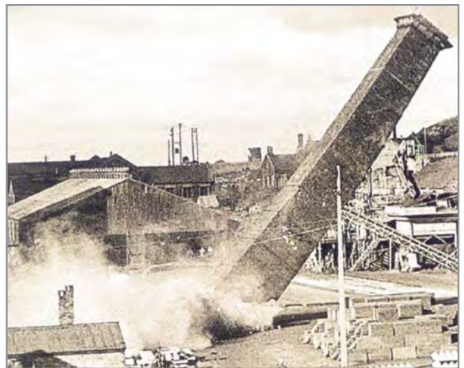
Demolition of Snedshill Trading Estate begins, 1967
