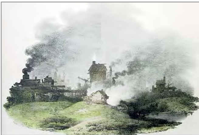
Snedshill Iron Works (later Priorslee Furnaces), c.1821
