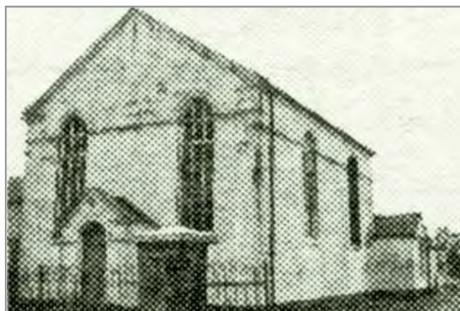
Sneds Hill Methodist Chapel, demolished for housing, 1988
