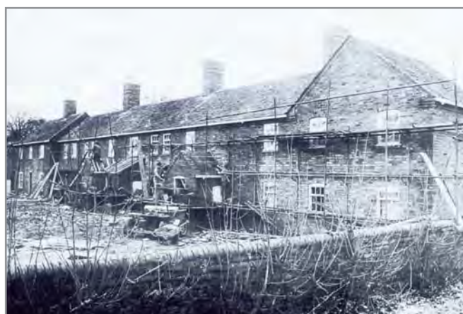
Stable Row undergoing reconstruction, 1977
