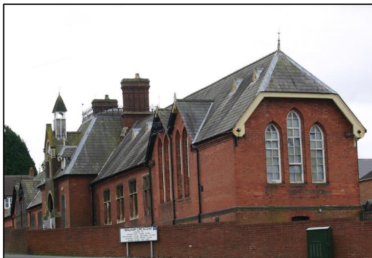
The Gower building currently stands empty and in a poor condition
